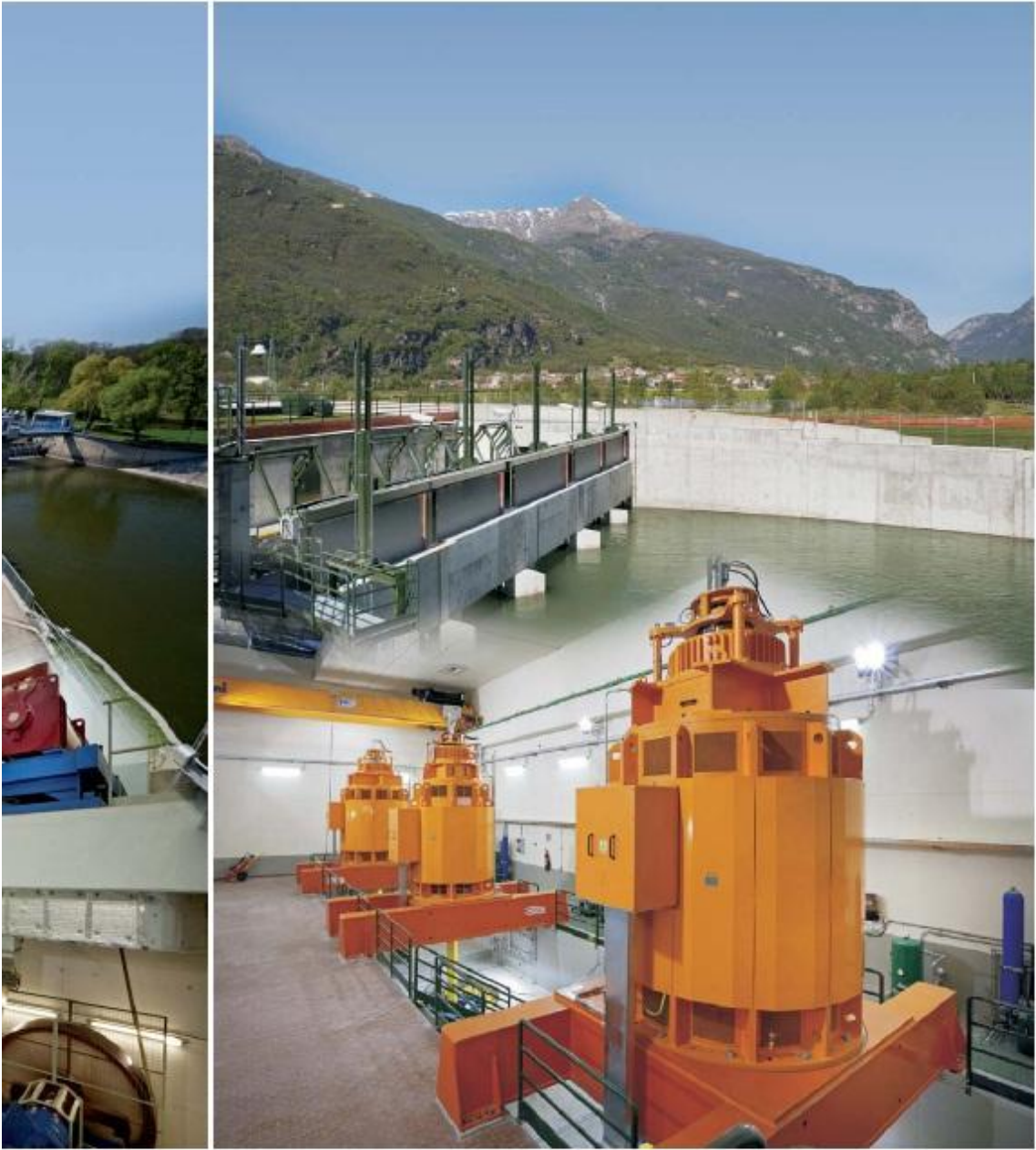
Montestrutto HPP Italy
