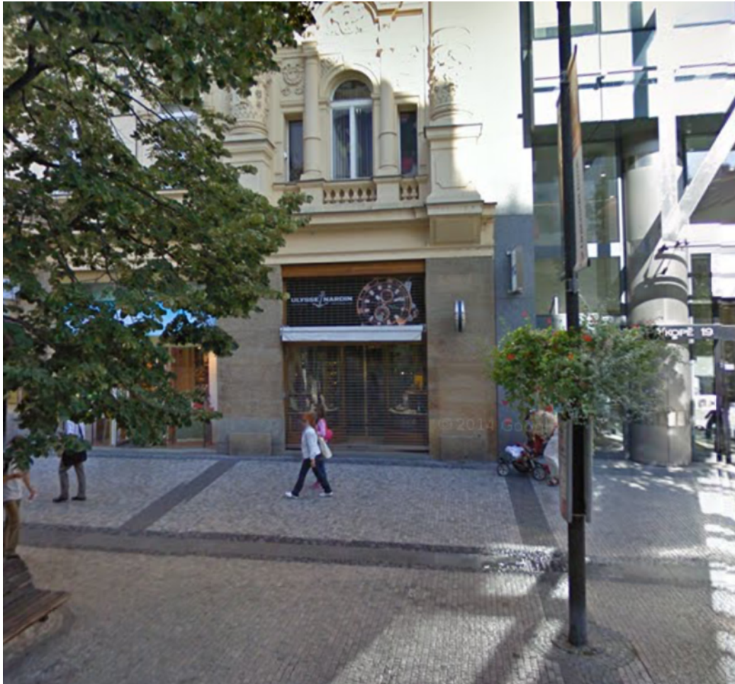
Obr. 12 Pohled z ulice [21]
