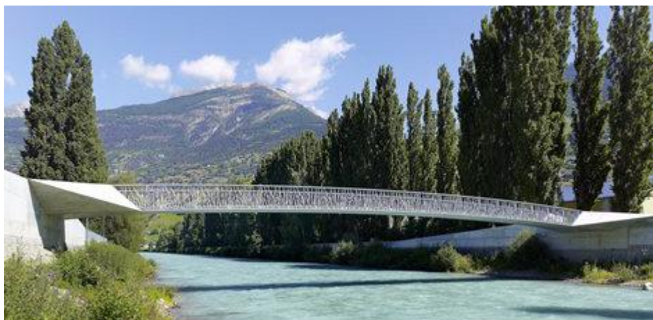
Obr. 66 The Footbridge Over The Vispa
