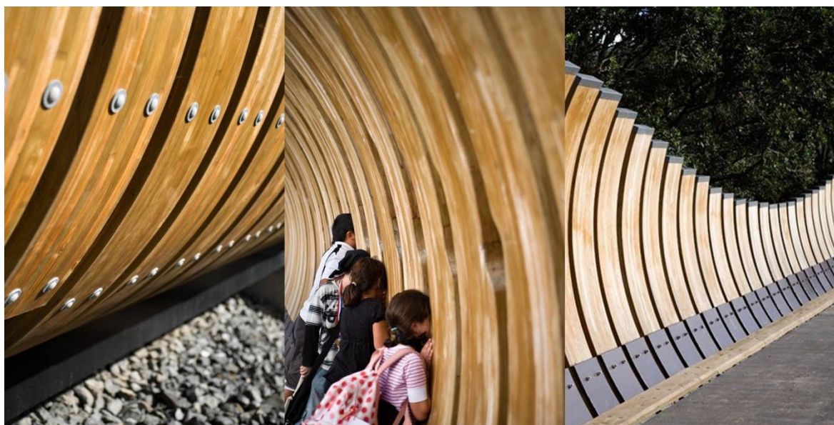
Obr. 65 The Onepoto Footbridge – detail
