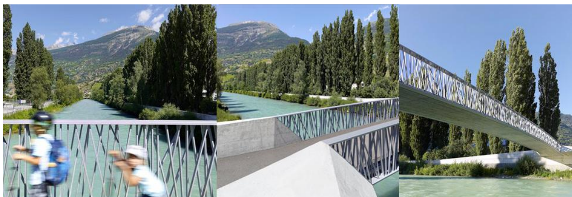
Obr. 67 The Footbridge Over The Vispa – detail
