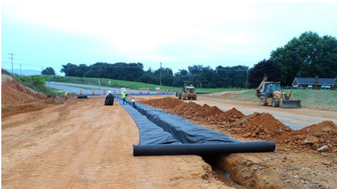
Figure 13 Practical use of geotextile (19)
